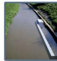
Water flow sensor testing
